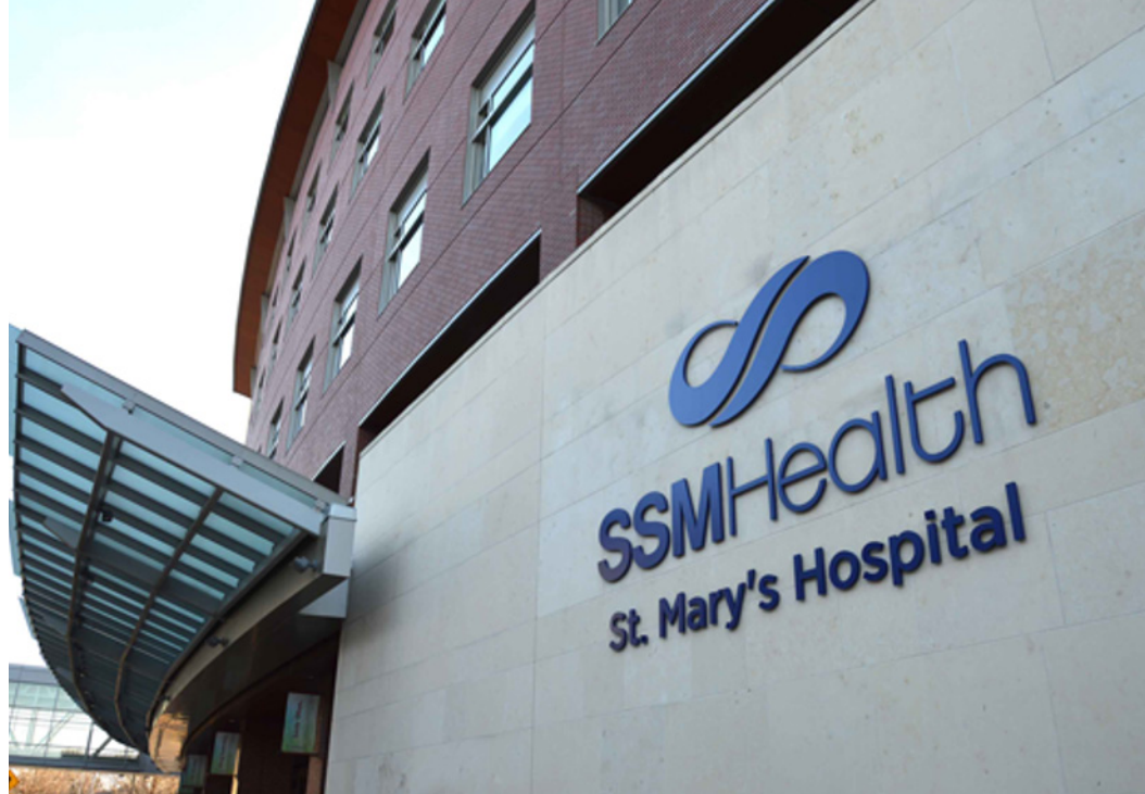
Above: Outside SSM Health St. Mary's Hospital in Madison, WI.
