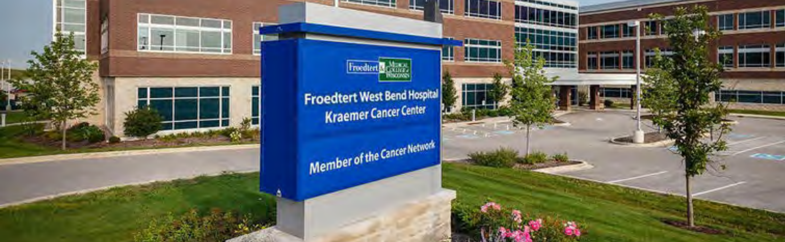
Below: Froedtert West Bend Hospital
